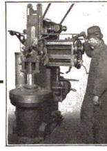
Boring and Turning the Casting
